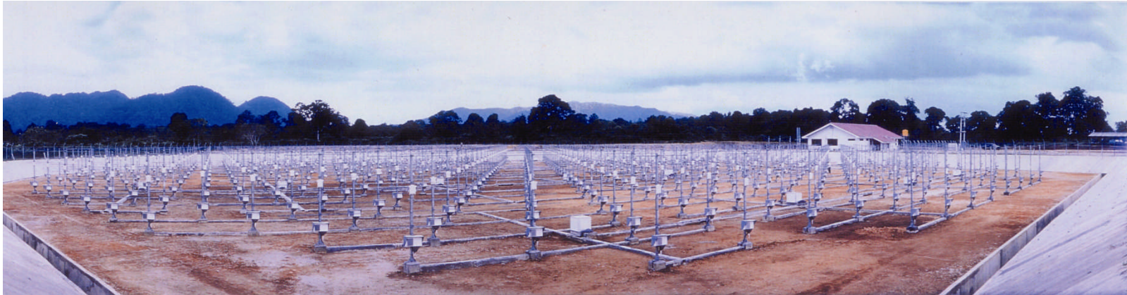
Antenna field (110m in diameter)
